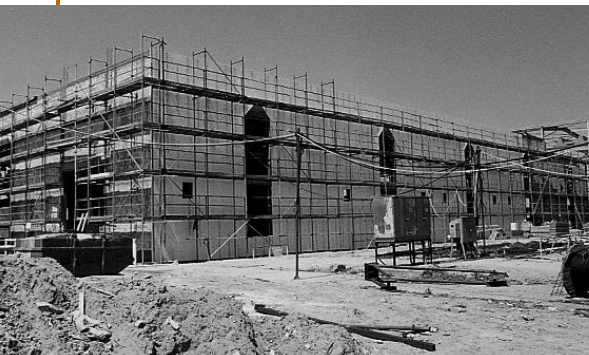
The new Training Centre under construction
